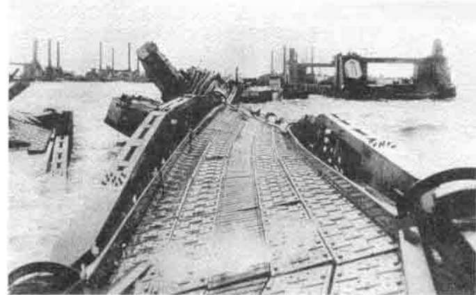
Following the storm of 19 June, 1944: the Mulberry under construction at Omaha Beach was a twisted wreck.
